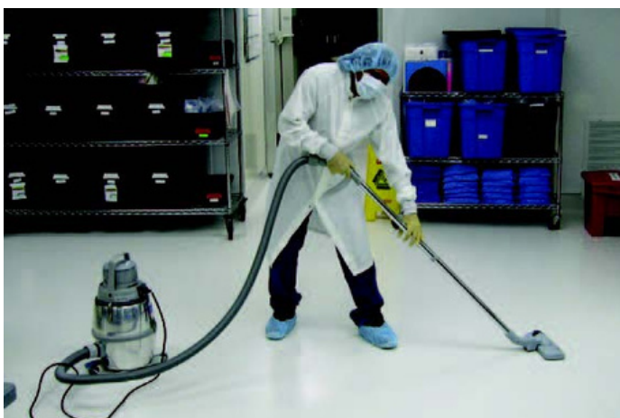
Figure 2: The first step in the cleaning process should be to vacuum all accessible surfaces.
